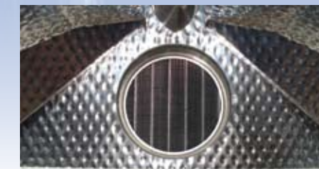
Water-cooled heat exchanger installed
